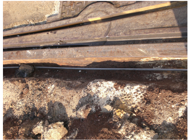
Figure 4. New Style Heater Installed
