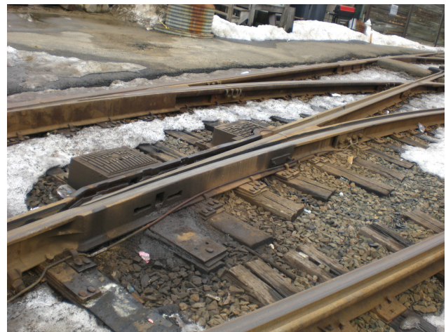
Figure 2. Heater Installation for Open Switch
