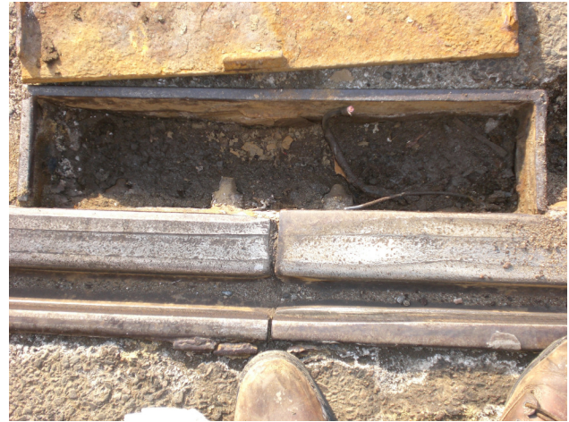
Figure 3. Pipe/Joint Box Configuration
