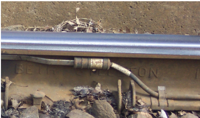
Figure 6. New Style Heater Terminal
