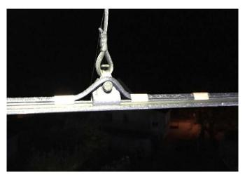
The heating cable is secured to the contact wire with phosphor-bronze attachment clips to avoid galvanic corrosion. The heating cable is in a triangular shape. This makes it very easy to mount on top of the contact wire and the shape provides excellent thermal contact to the contact wire. Finally it also makes the fastening clips easy to handle and very efficient to mount.
